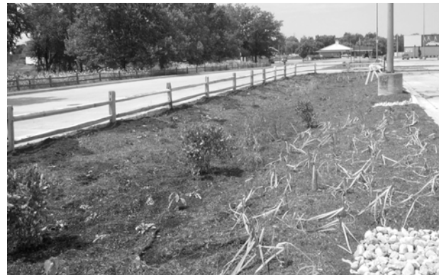
Finished raingarden near Shiawassee River, along Jerome St. © Andrea Berry, SCD.
